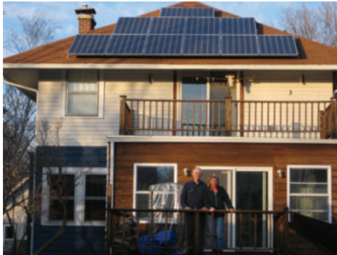
A view of the solar panels on the rear roof; the rest of the panels are on the southern side of the house.
